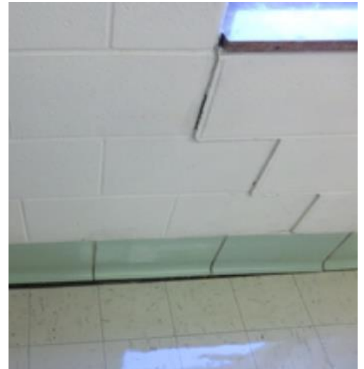
Diagonal Cracking/Separation between Floor and wall
